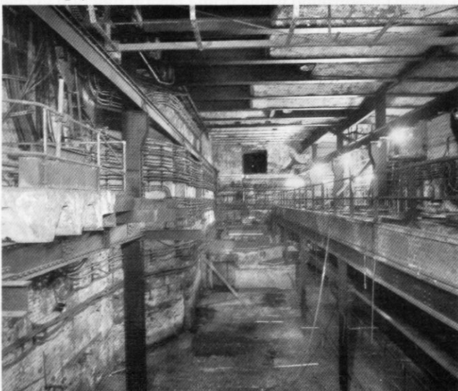
Embankment substation chamber in 2008. Photo Nick Catford
